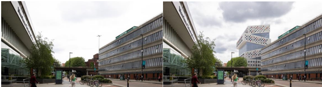
View 4: Existing and proposed view from footway on eastern side of Oxford Road adjacent to Manchester Technology Centre looking south.
