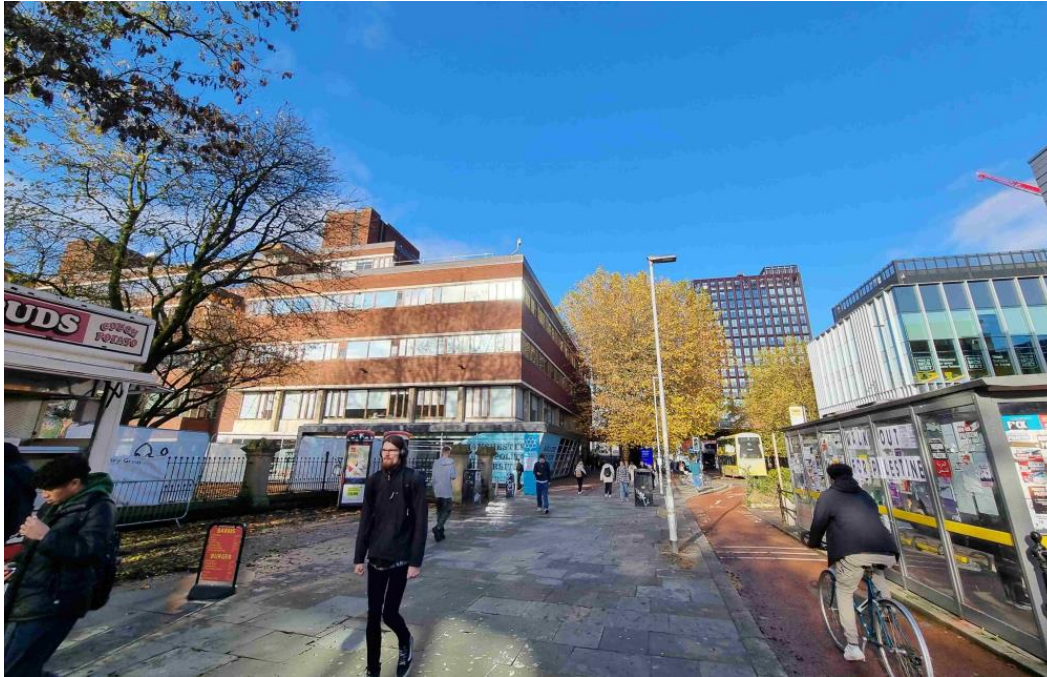
All Saints Building as seen from Oxford Road travelling northwards
